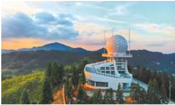
204 图 5 闽侯 S 波段双偏振相控阵天气雷达 205 Figure 5. Minhou S-band Dual-Polarization Phased Array 206 Weather Radar
