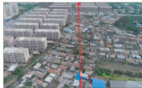
图 9 龙卷穿过义和村,擦过瑞福居小区,移向尚品铭城 Fig. 9 The tornado's passing through Yihe Village, skimming Ruifu Community and moving to Shangpin Mingcheng Community
