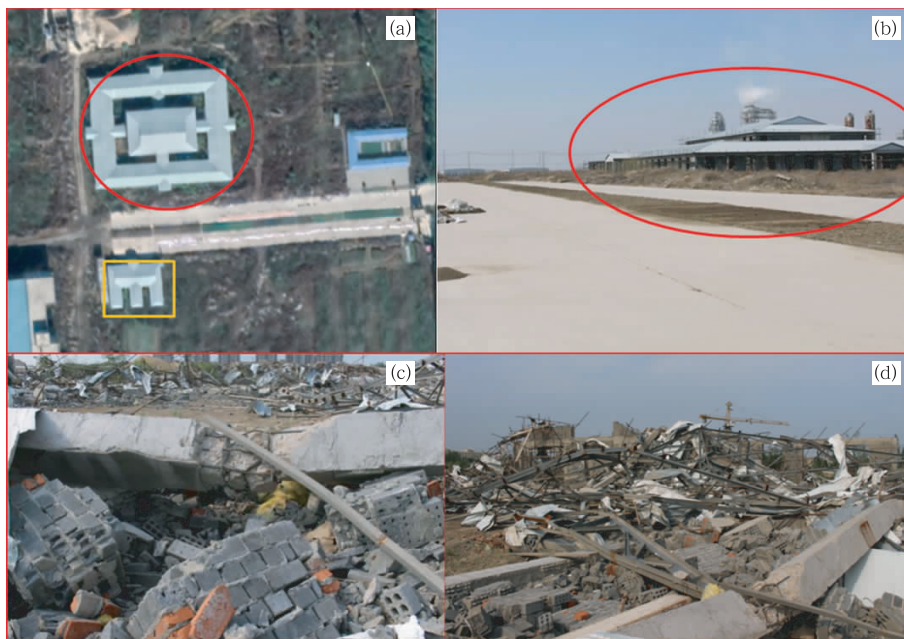
图 12 图 11 中食堂灾前顶视(a)及平视照片(b),灾后钢筋混凝土框架结构几乎被夷为平地(c,d) Fig. 12 Top view (a) and horizontal view (b) of canteen in Fig. 11 before disaster, and reinforced concrete frame structure almost flattened after disaster (c, d)
